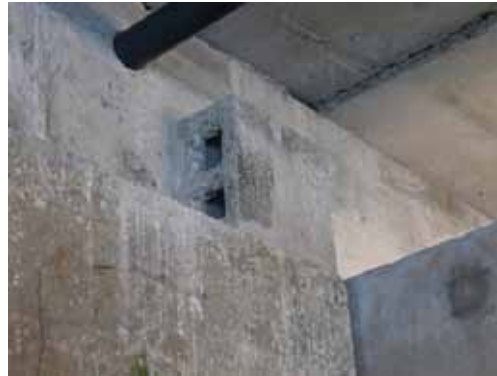
Figure 5 One of the 27 Central Pier breeding chambers. Each entrance is about 15cm square with a depth of about 60cm. Black Guillemots consistently use the lower hole as they have a platform provided by the top of the pier pillar upon which to land; they have never used the upper hole
