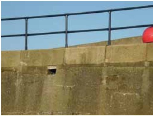
Figure 4 One of the 15 North Pier nesting holes. Each hole has a square profile of about 30cm x 30cm and is about 100cm in length. Some of the slightly larger holes (like the one illustrated) have a reduced entrance to lessen predation by Hooded Crows Corvus cornix and Herring Gulls Larus argentatus
