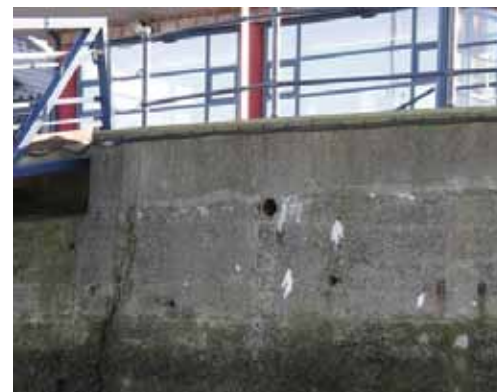
Figure 7 One of the six South Pier breeding holes; each hole has a diameter of about 15cm and a length of about 120cm
