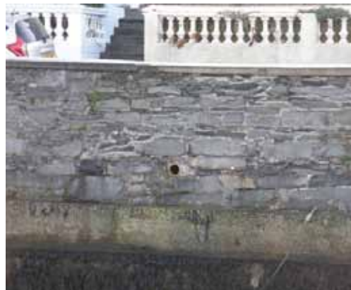
Figure 9 One of the Long Hole breeding tubes. Each tube is about 20cm in diameter and about 100 cm in length. The masonry around some of the tubes has decayed and some birds use that space instead leaving them very exposed
