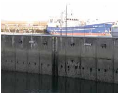
Figure 6 The marina face of the Central Pier showing plastic breeding tubes and wooden boxes. The plastic tubes have a diameter of about 25cm and are about 120cm long; they are open at one end only. The wooden boxes are described in detail in Leonard et al. 2015
