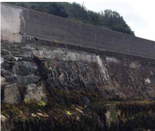
Figure 40 An example of artificial nest sites in the sea wall along Lough Shore Road.
